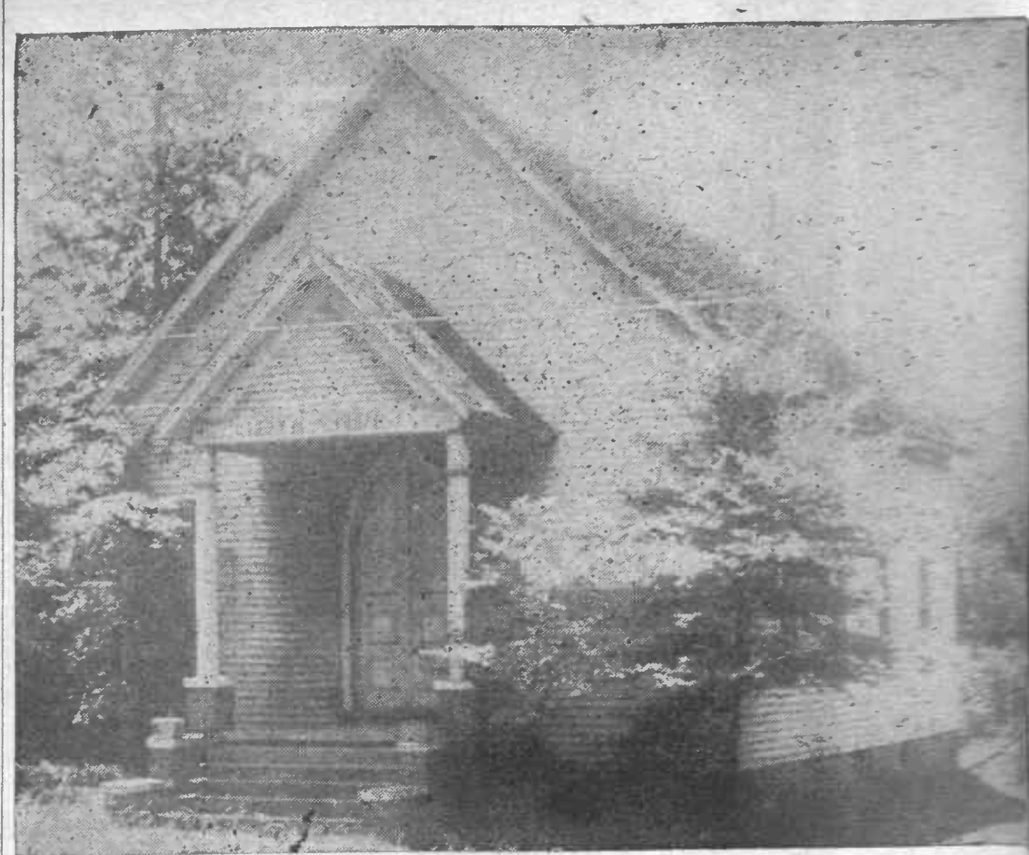
IUKA CHURCH OF CHRIST—This building was raised about 1948 and much of the heavy timbers salvaged from the old building was used in the new Church. The doors at the entrance of the building, once pointed at the top were cut off straight and re-finished for the present building. It stands on the same lot located on Eastport between the Perry Kimberly residence and the home of Mrs. Mary Massey. The congregation then numbered about twenty-five. Today the membership is over one hundred.
